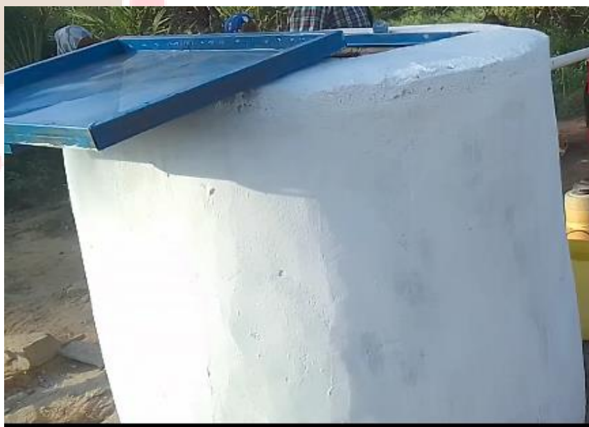
Representation of the expected borehole protection chamber
